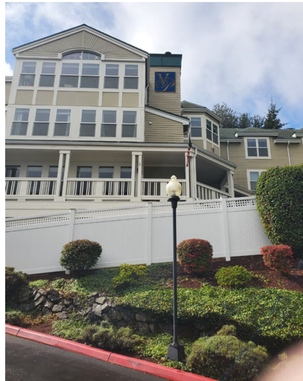
Proposed Install Location - Details Pending Survey
